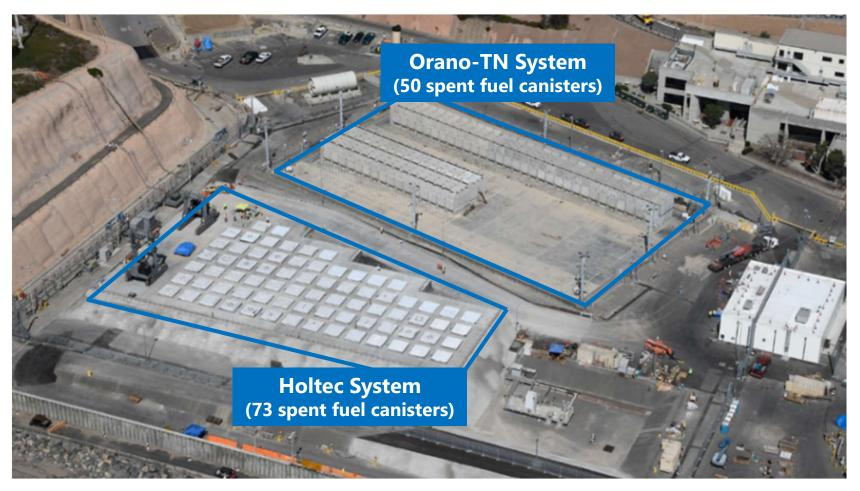
**Provides Passive Dry Cask Storage for Spent Fuel While On Site**
