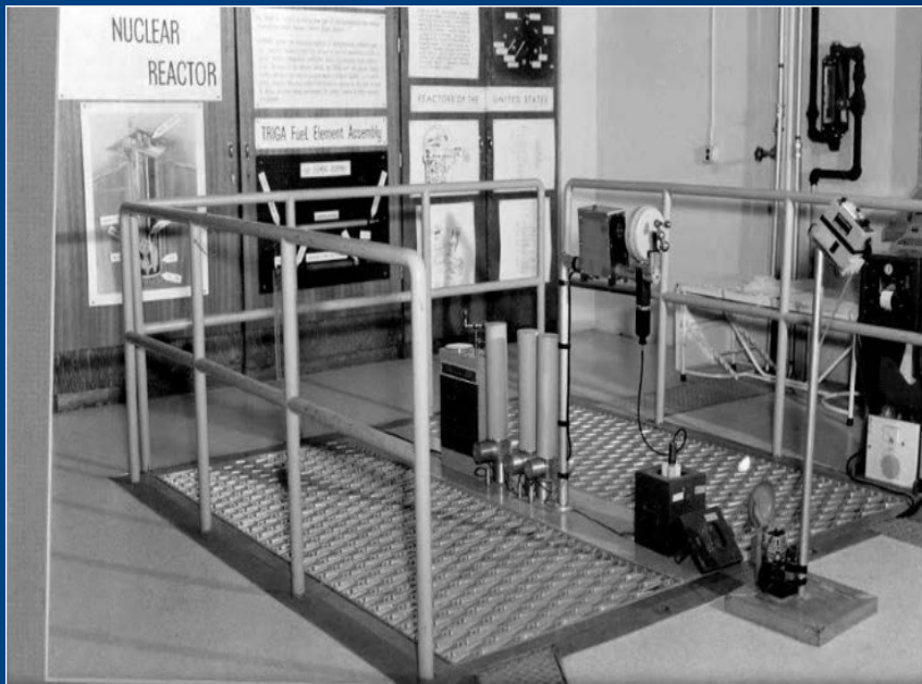
Veteran Administration Hospital TRIGA 18 Kw Reactor Facility
